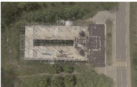
Figure 3: Orthomosaic image of Bachelor residential building of Southern Campus
